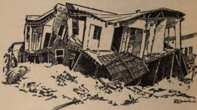
FIG. 85. — House wrecked in San Francisco earthquake of 1906 because the floors and partitions were not securely fastened to the walls (after R. L. Humphrey).
